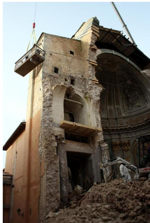
Fig. 11. Cathedral of L'Aquila and installation of sensor nodes via a basket hanging from a crane
