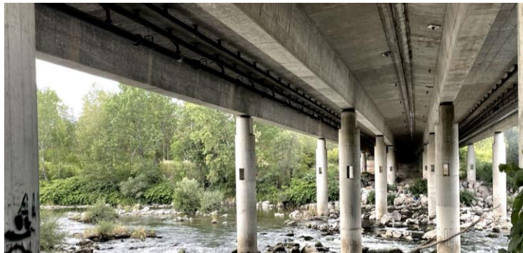
Fig. 5. Underside of the bridge at the crossing of the Sava river
